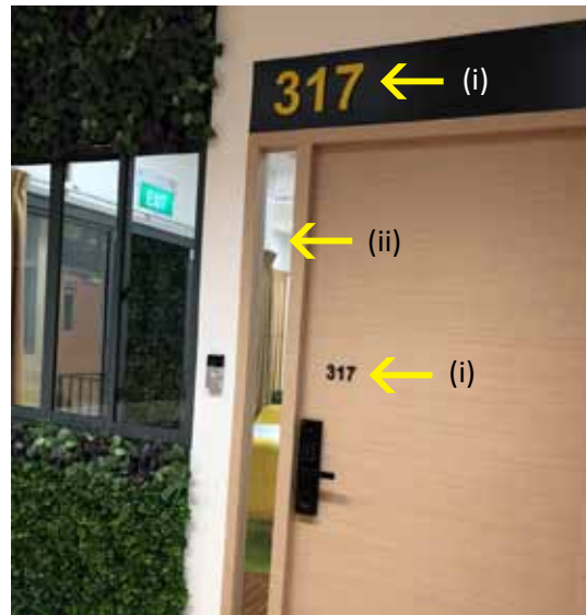
Photo 5: (i) Unit number; (ii) See-through side panel at the main door (indicated by yellow arrows)
