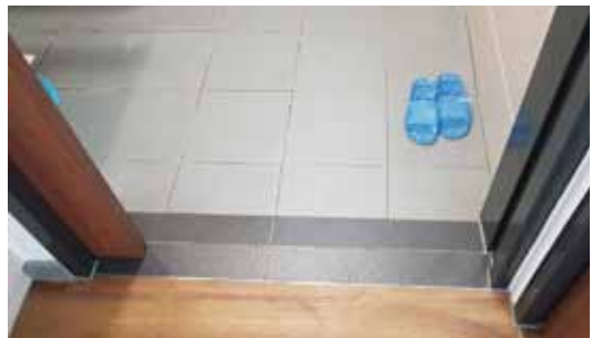
Photo 13: Ramp at the bathroom-toilet entrance
