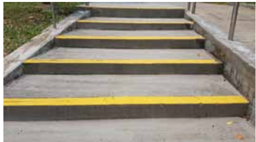
Photo 32: Steps marked with yellow paint/ strips (I'DGO 2014)
