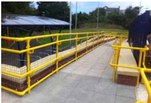
Photo 30: Handrails along the ramp (source: https://www.roofedge.co.uk/news/story/access-for-all-with-key-access-fittings )
