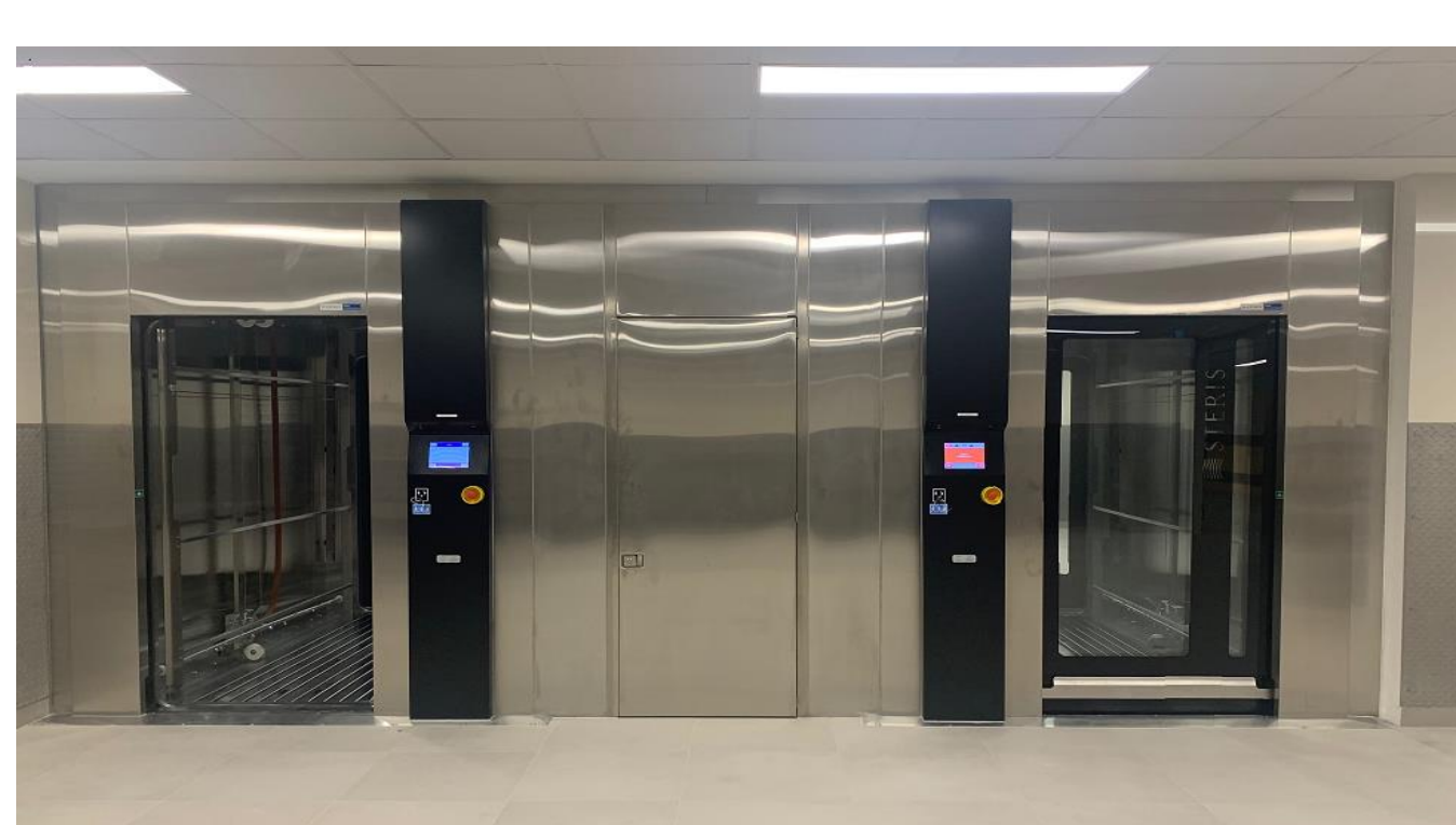
Cart washer disinfector at B2 SingHealth Tower
