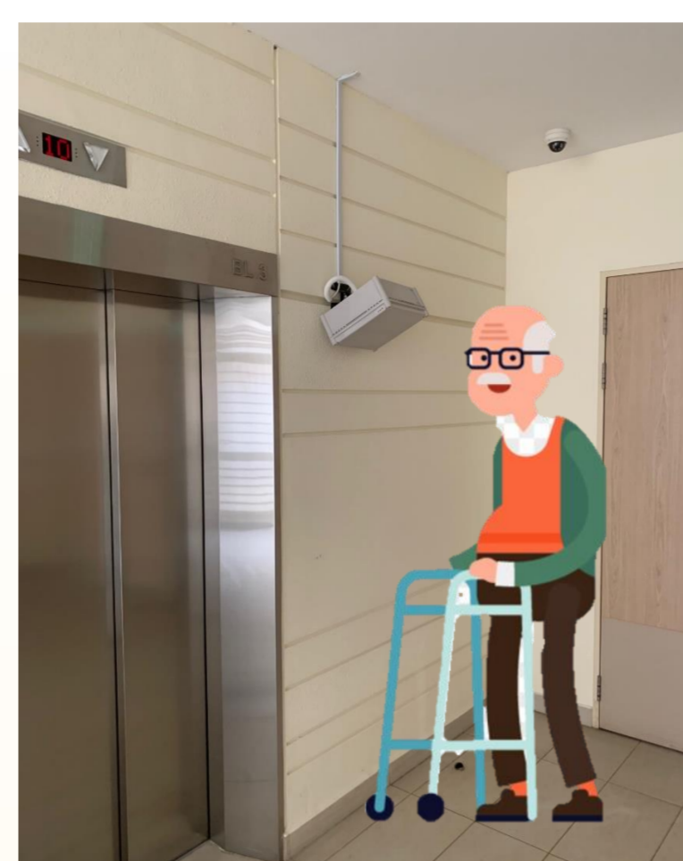
Resident moves past a RFID reader at non-permitted area (e.g. lift lobby)
